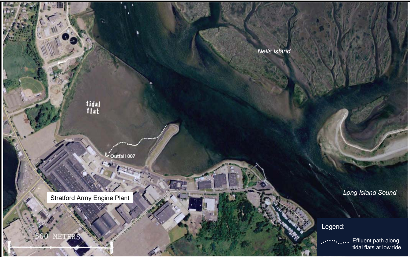
Figure 2-11b Low Tide Effluent Path
