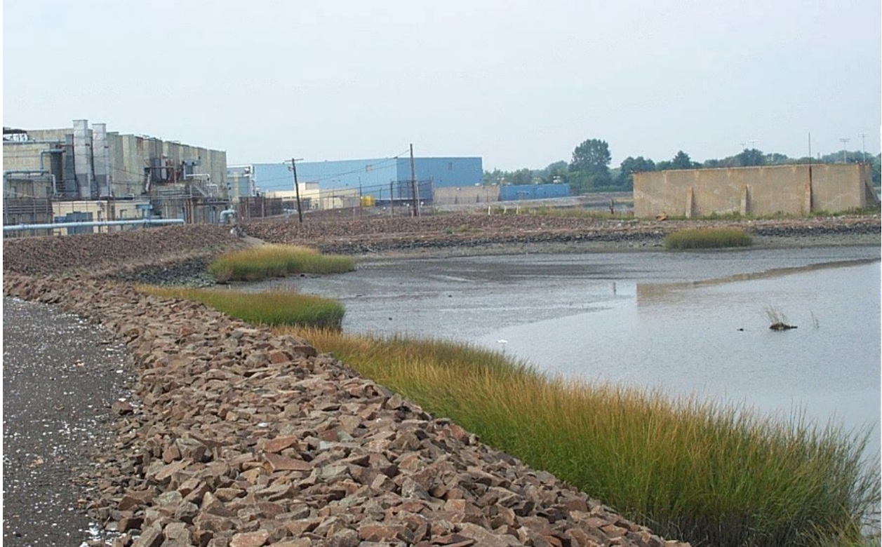
Figure 0.1. Photograph of SAEP (left) showing the causeway extending toward the Housatonic River (right). (Photograph by Durgin on 9/24/01).
