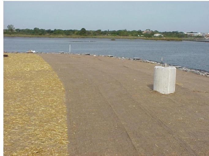
30. Looking north along Causeway with final grading, jute mat application and straw mulch, (photo courtesy of R. F. Weston).
