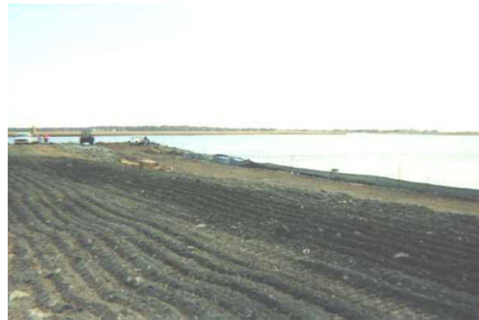
12. Scarification and grading of lower cover system "acceptable" fill material on upper cover area to achieve subgrade contouring.
