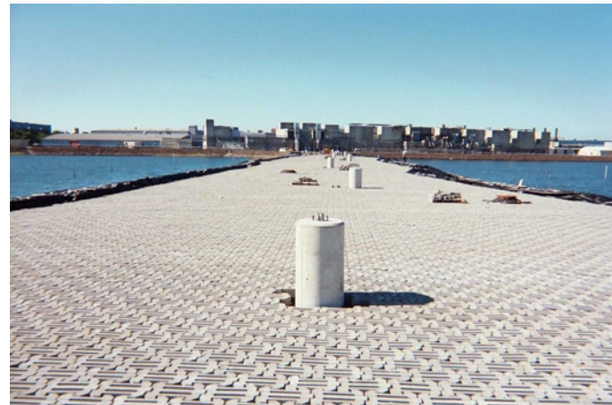
28. Completed articulating concrete block deployment prior to placement of interstitial gravel fill, (photo courtesy of R. F. Weston).
