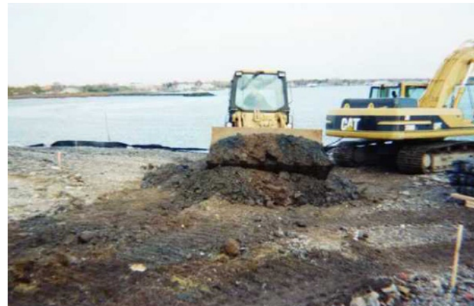
8. Relocating subgrade spoil excavation from lower cover system for scarification and drying.
