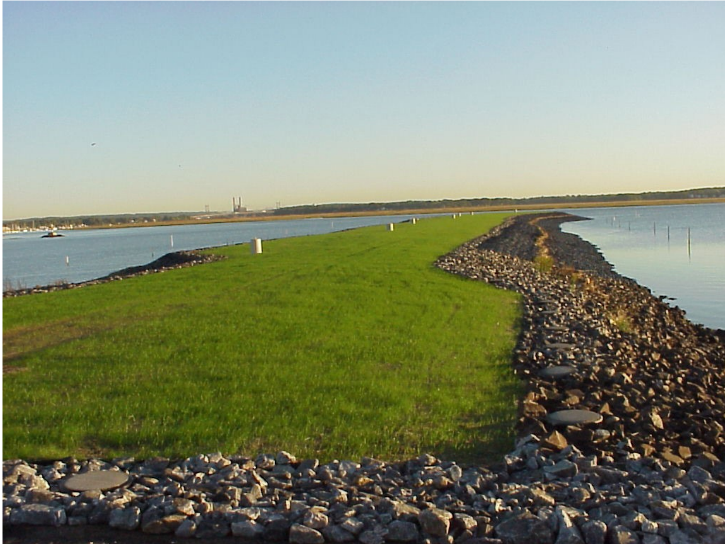
33. View of Causeway with established vegetative cover post-construction (Oct 2002), (photo courtesy of R. F. Weston).
