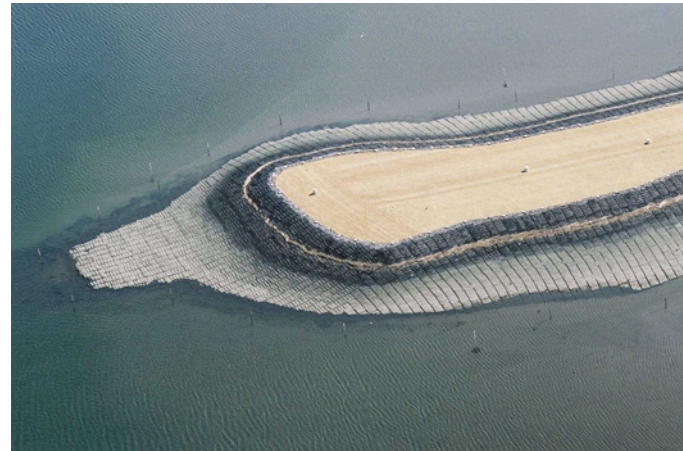
32. Aerial view of Causeway tip post bedding sand application. Note grayish color of marine mattresses indicating algae growth, (photo courtesy of R. F. Weston).
