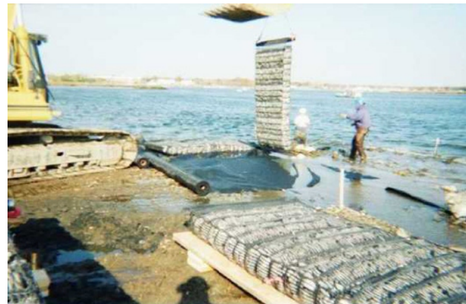
4. Marine mattress deployment at low tide (looking north towards Housatonic River channel).
