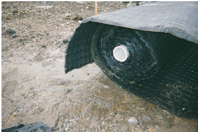
7. Reinforced geogrid utilized under riverine sediment/causeway fill interface details to provide support for marine mattresses.
