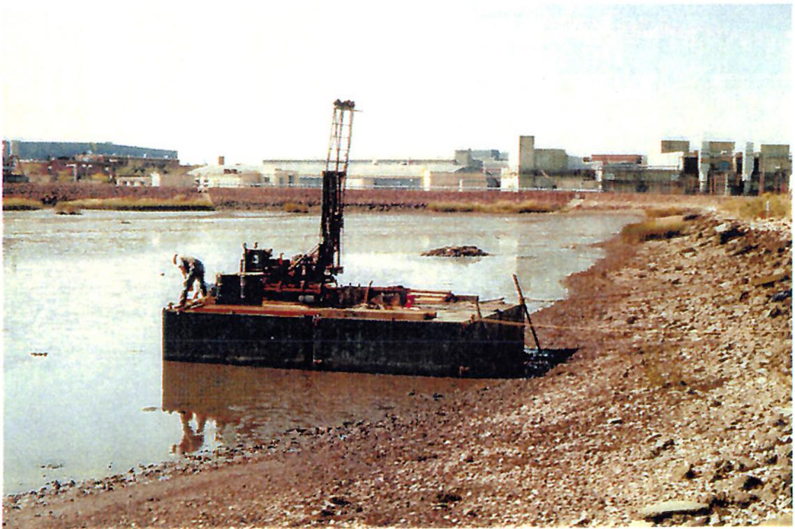
**Picture # 10** The barge rig is set up at GB-00-05, with one edge of the barge just touching the Causeway fill material. The view is toward the SAEP facility, and shows full exposure of the mud flats at low tide.
