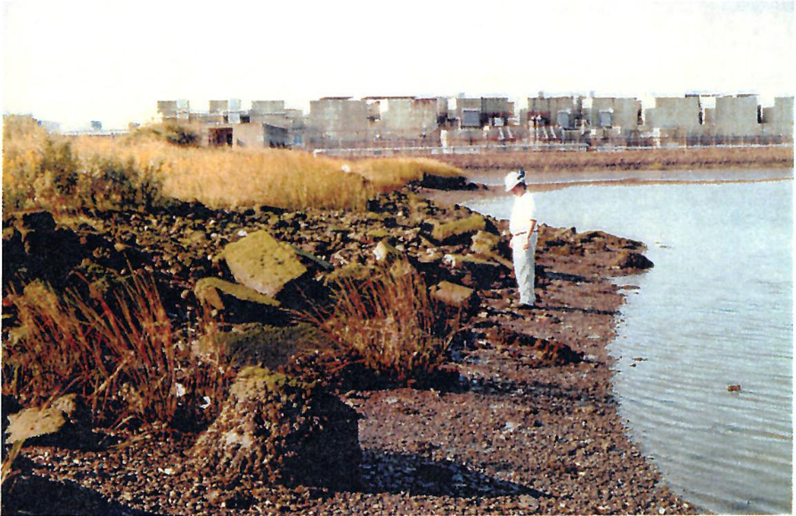
**Picture # 7** Example of the variation of the fill material that was deposited along the western side of the Causeway.
