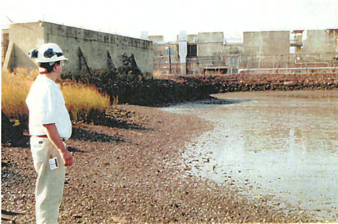
**Picture # 4** At low tide conditions, looking toward the SAEP facility, with Bldg. # 59 on the left. Note the high tide mark coloring the rip-rap in the distance. Also note the contact of the filled material of the Causeway with the mud flat sediments, the contact represented by the "wetter" mud flat soils.
