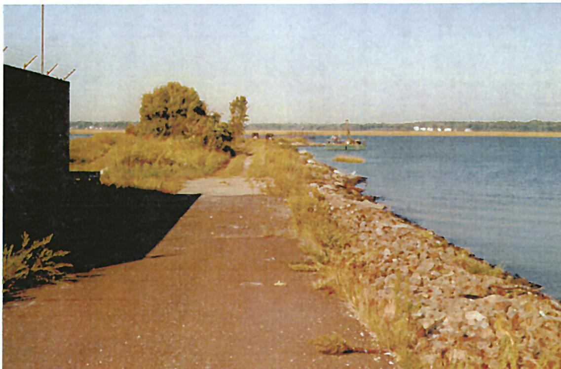
**Picture #1** Looking northerly down the length of the Causeway, with Bldg. # 59 at the left. Bituminous concrete pavement gives way to dirt just beyond Bldg. # 59. Barge rig is set up at GB-00-05. Water is near the mean high tide mark.
