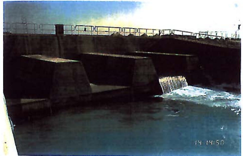
Photo 6: Jebel Ali "G" water outfall
