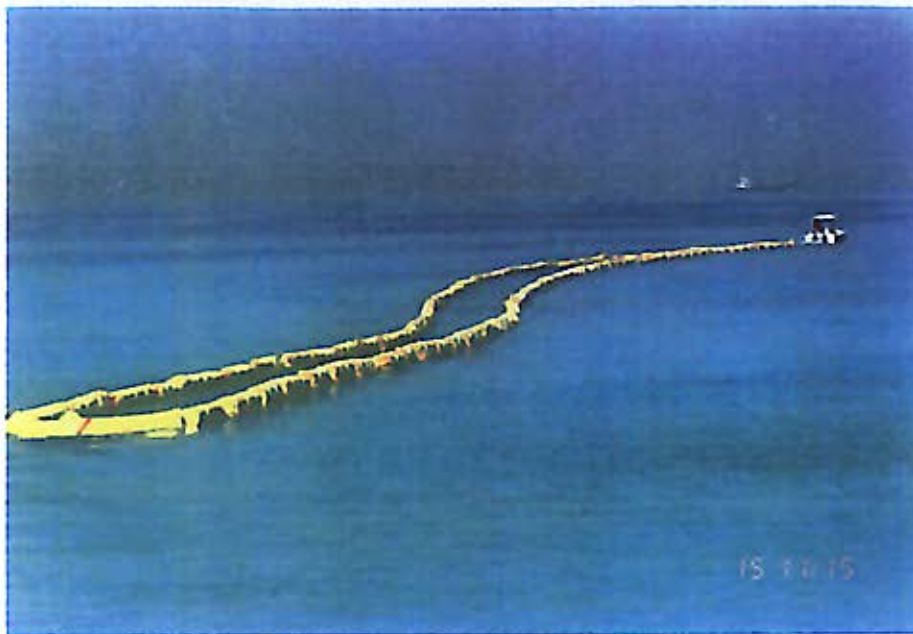
Photo 7: Towing SeaCurtain Boom to Seawater Intake site
