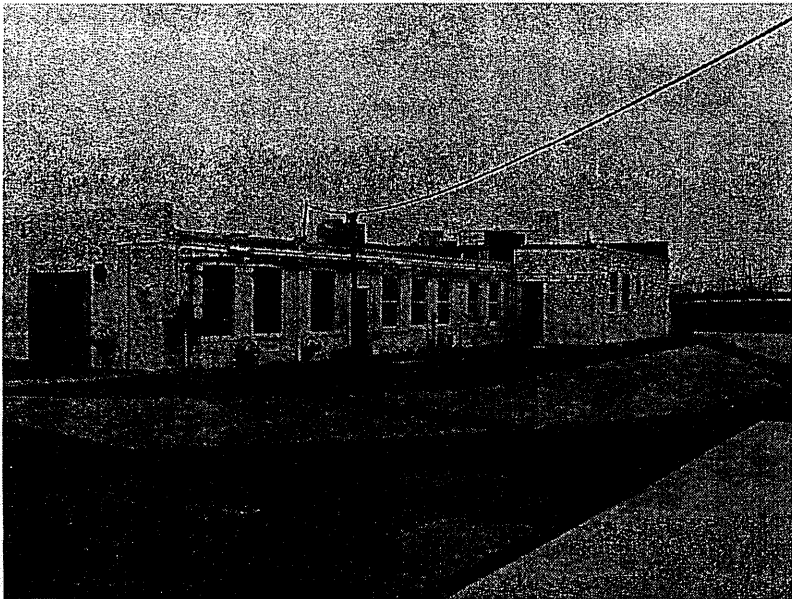
Overview of building from Southeast
