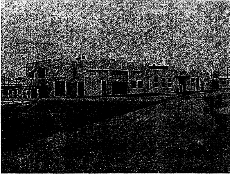
Overview of building from Northwest
