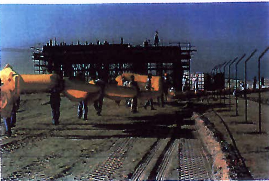
Photo 3: Moving Boom to Launch Site
