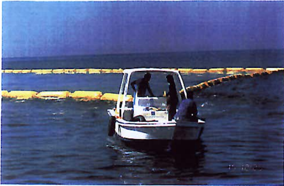
Photo 9: SeaCurtain Boom positioning around Seawater intakes
