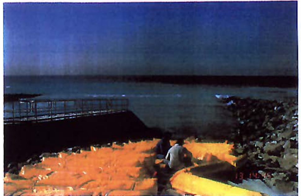
Photo 4: Positioning Boom on Boat Ramp for launch
