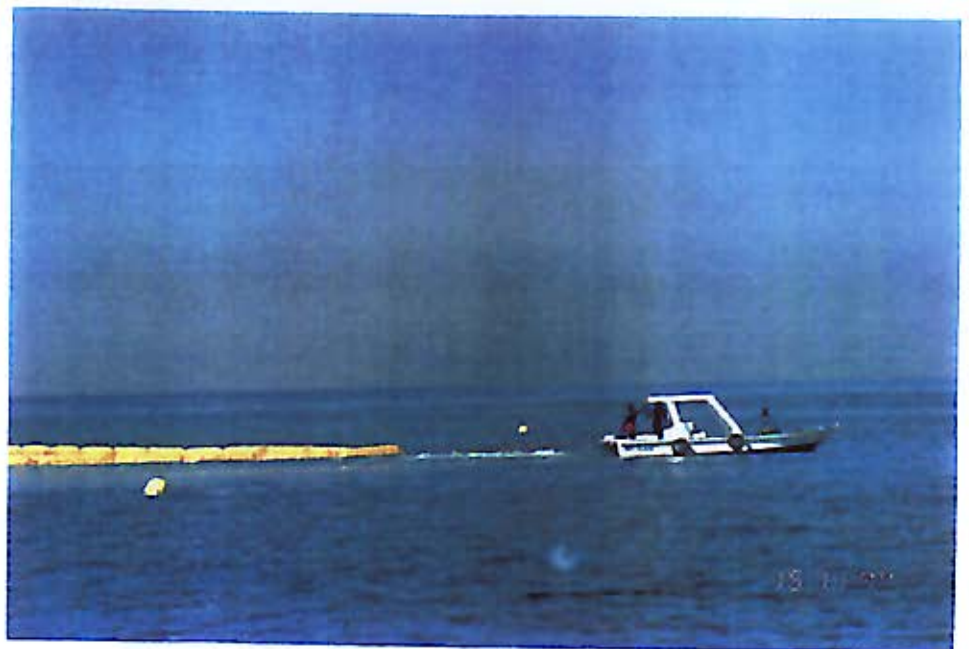
Photo 8: Positioning Boom around Seawater Intakes
