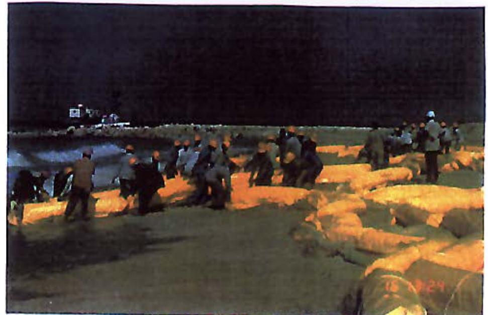
Photo 20: Removing SeaCurtain Boom from surfline
