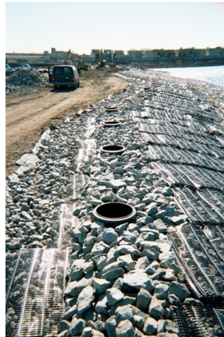
18. View of deployed marine mattresses to the north and east on the Causeway tip. Note Sea grass windrow and algae accumulation on mattresses.
