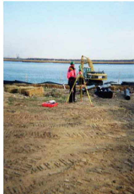
10. Survey of causeway and intertidal settlement/heave monitoring platforms.
