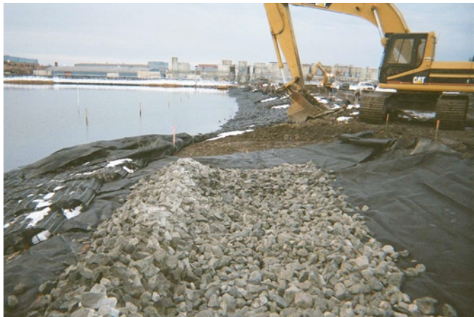
17. Rock filled transition between upper and lower cover systems.
