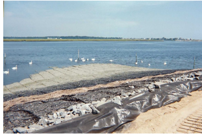
18. View of deployed marine mattresses to the north and east on the Causeway tip. Note Sea grass windrow and algae accumulation on mattresses.
