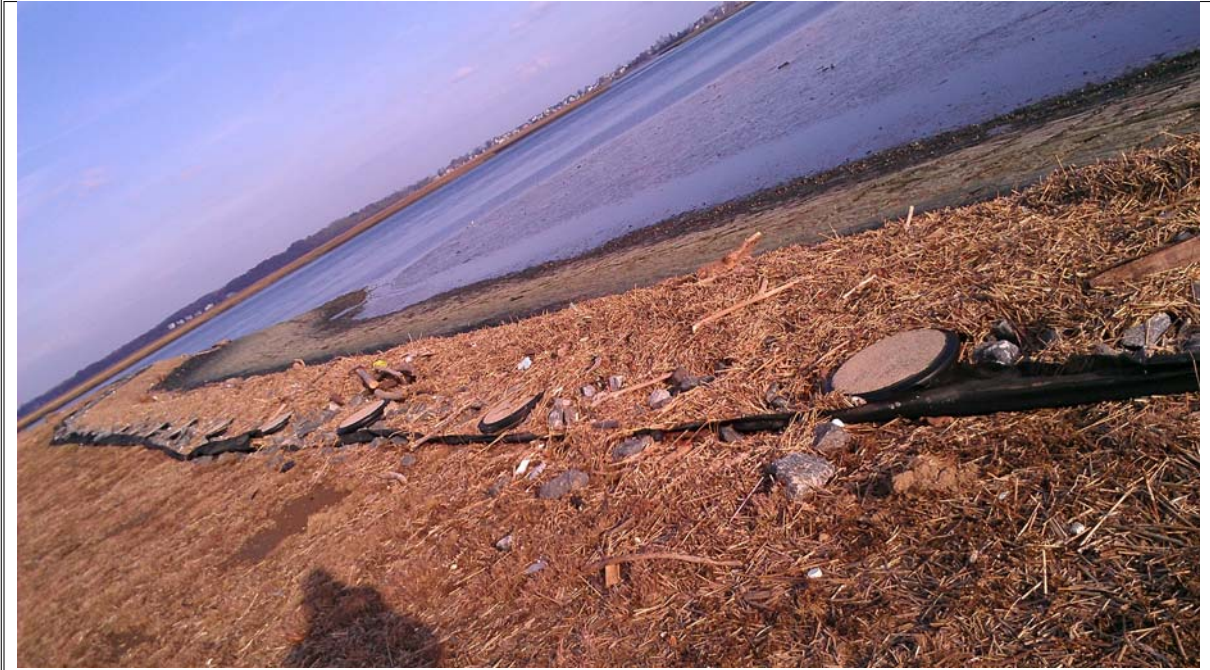
Photograph 7: Transition between upper and lower cover system, geotextile exposed adjacent to fence post base
