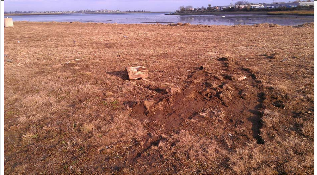
Photograph 35: Vegetative cover on causeway showing typical bare spots
