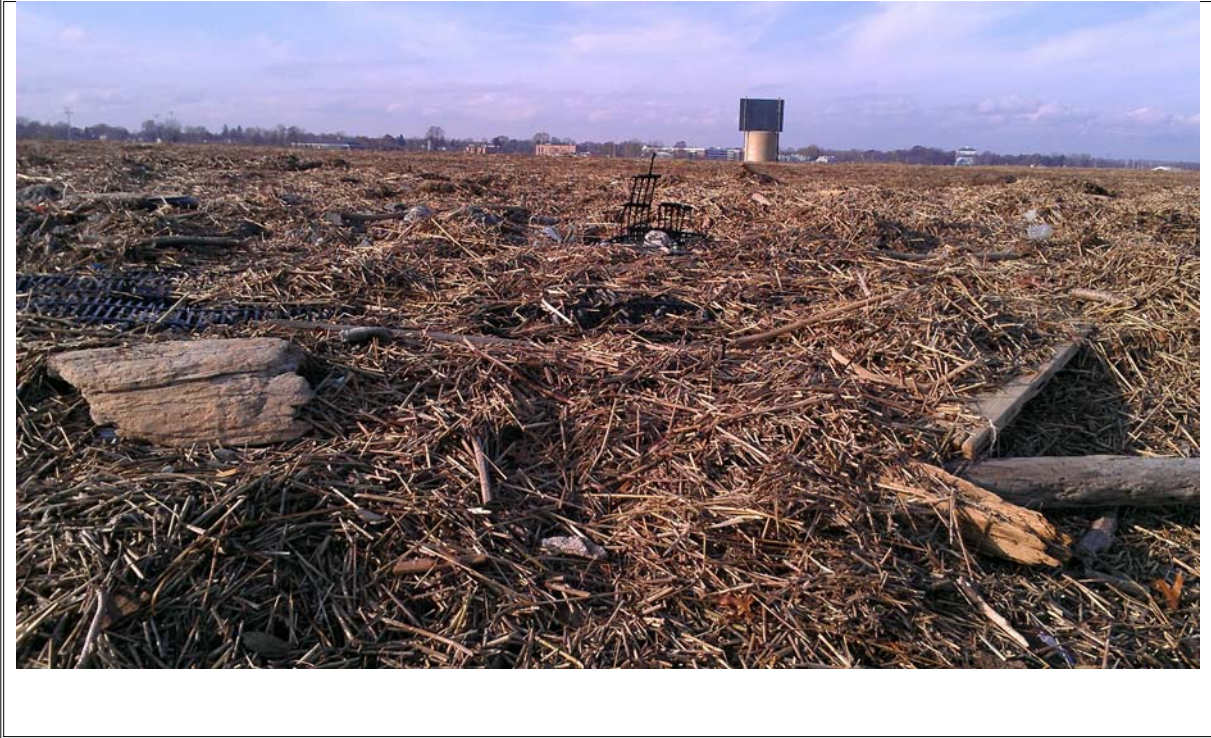
Photograph 33: Top of eastern side of causeway showing storm debris and vegetation condition
