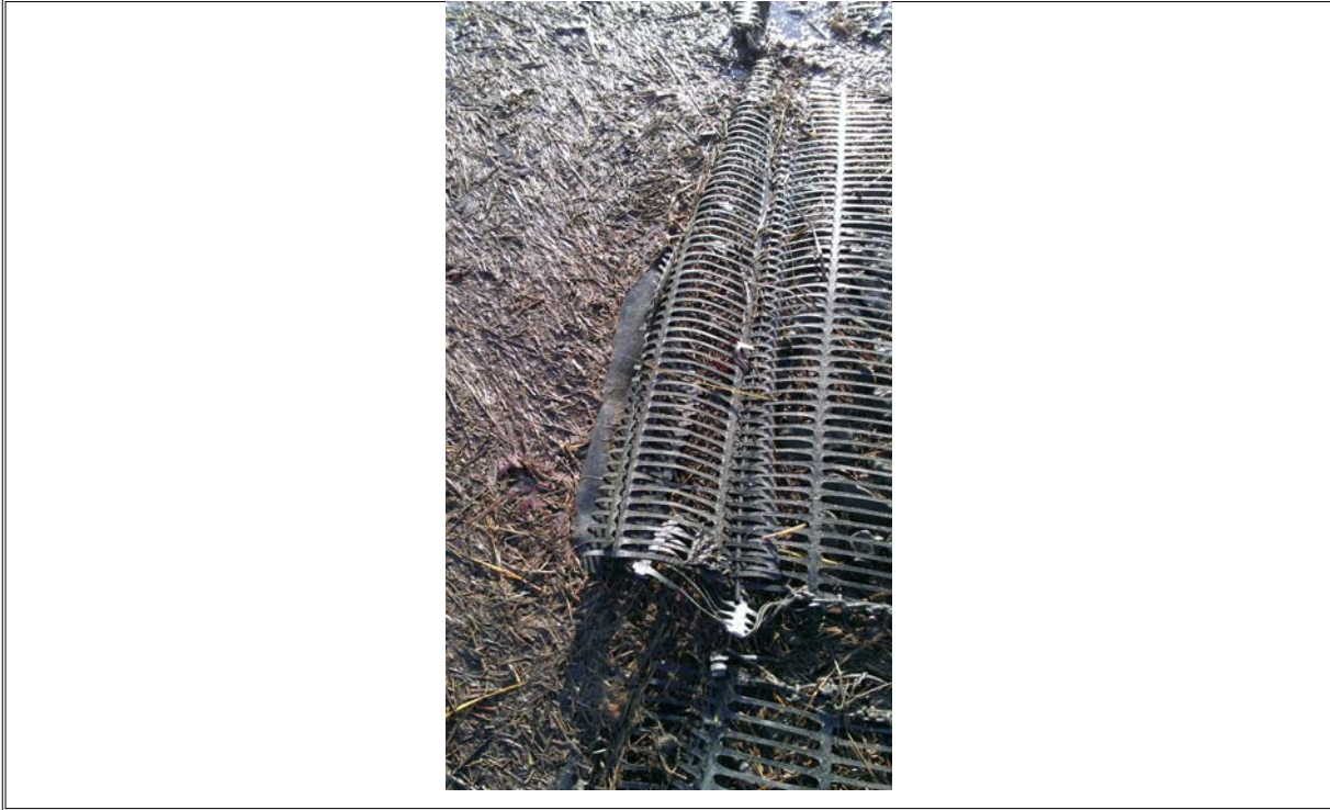
Photograph 11: East face of causeway showing marine mat edge
