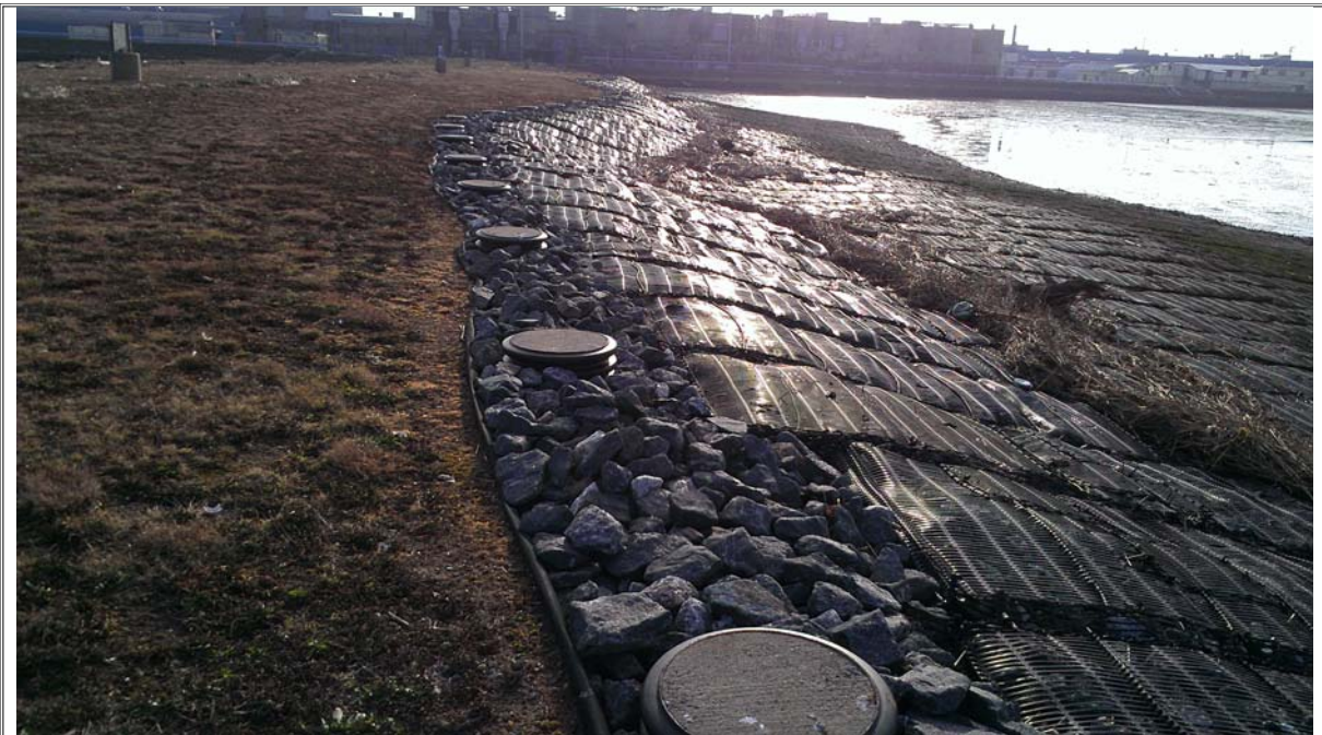
Photograph 35: Vegetative cover on causeway showing typical bare spots
