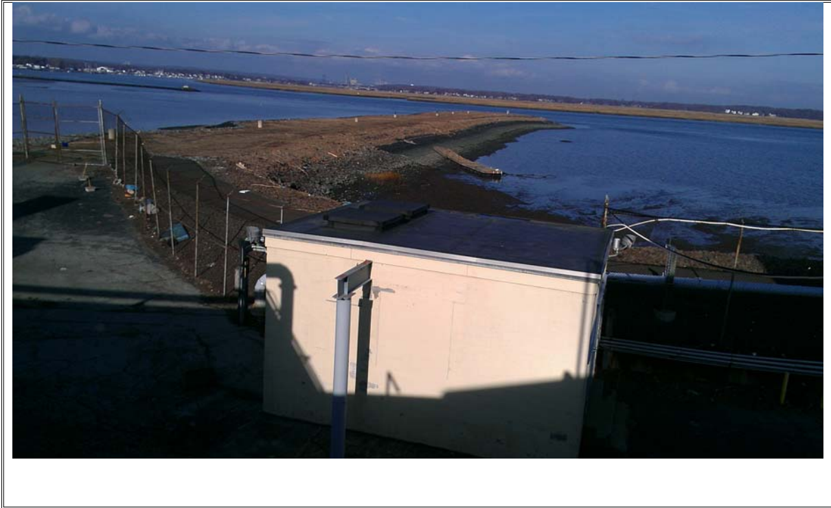
Photograph 3: Southwest face of causeway, view to north
