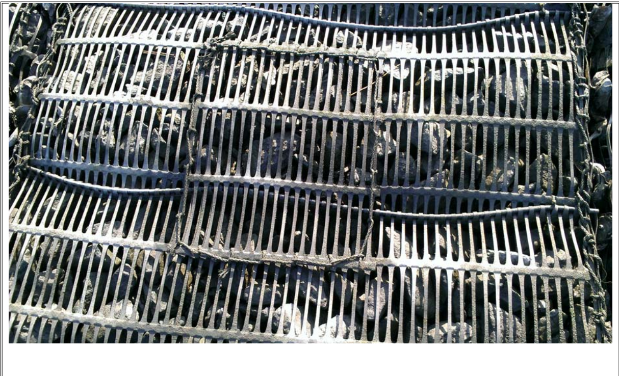
Photograph 20: Marine mat at eastern tip of causeway showing typical condition
