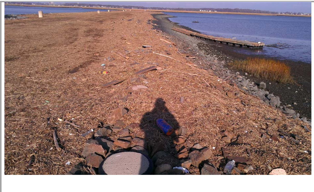
Photograph 6: Southwest face of causeway, view to northeast
