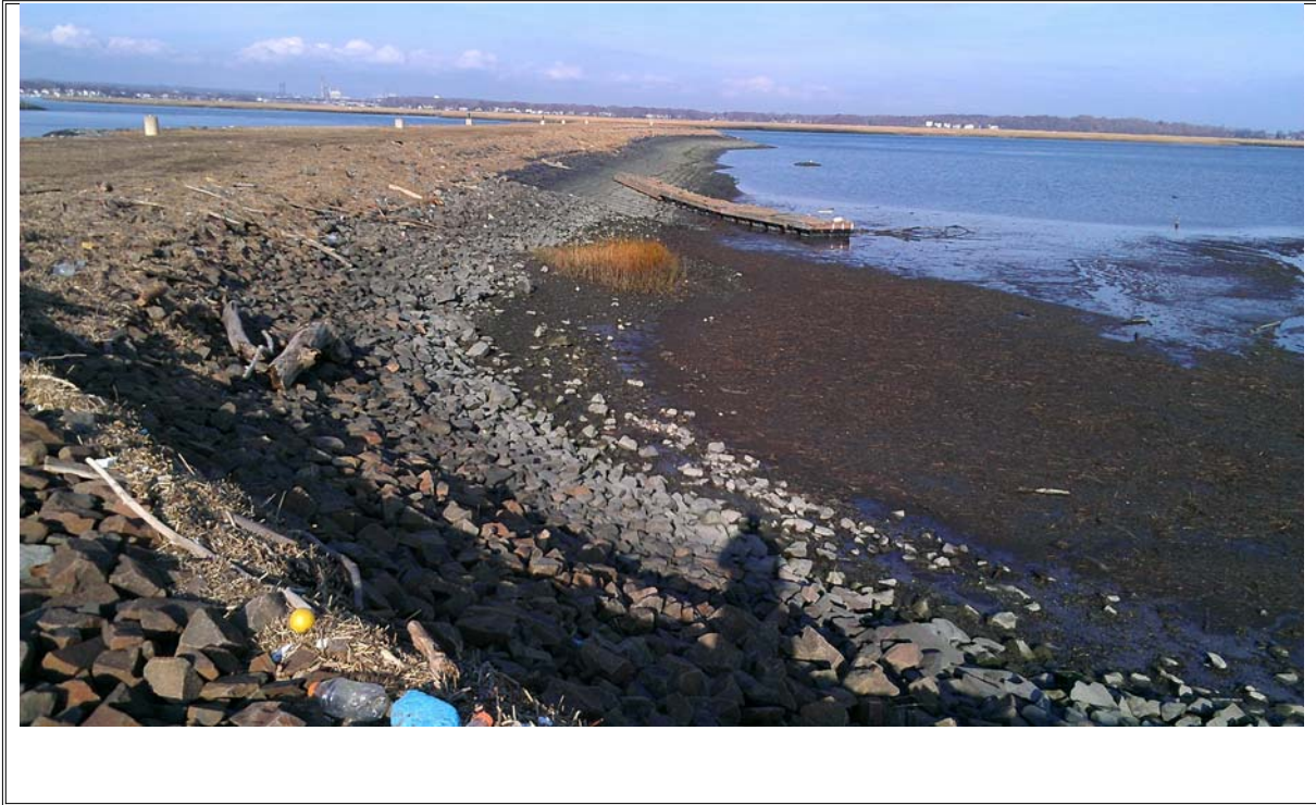
Photograph 5: Southwest face of causeway, view to northeast
