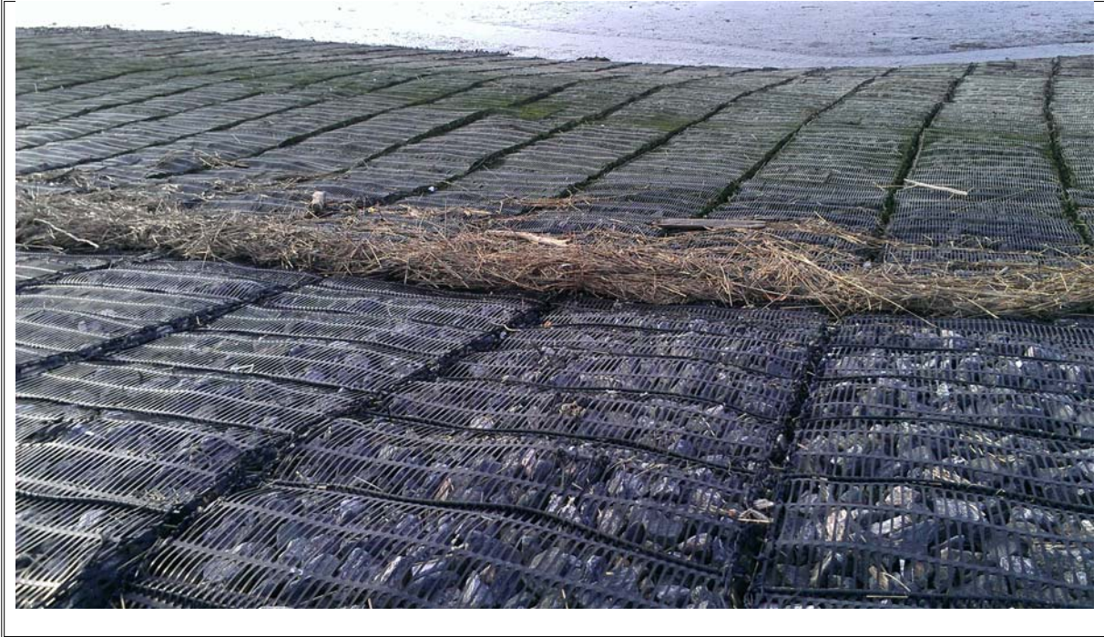
Photograph 25: View of west face of causeway, view to north
