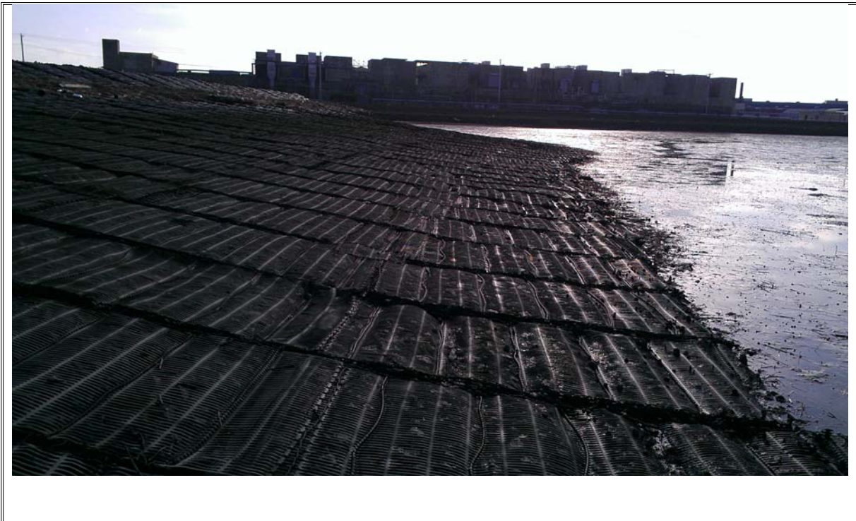
Photograph 26: Toe of marine mat slope, west face of causeway
