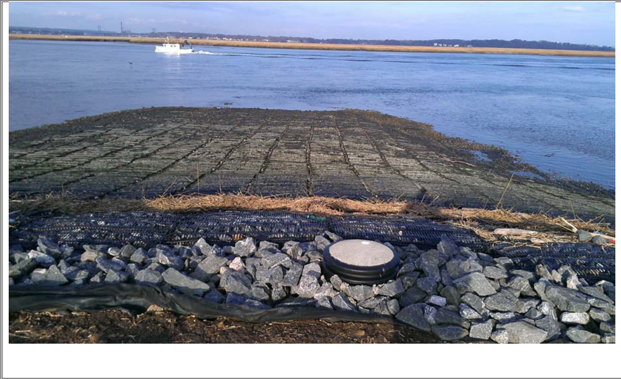
Photograph 21: Marine mat at eastern edge of causeway showing typical condition
