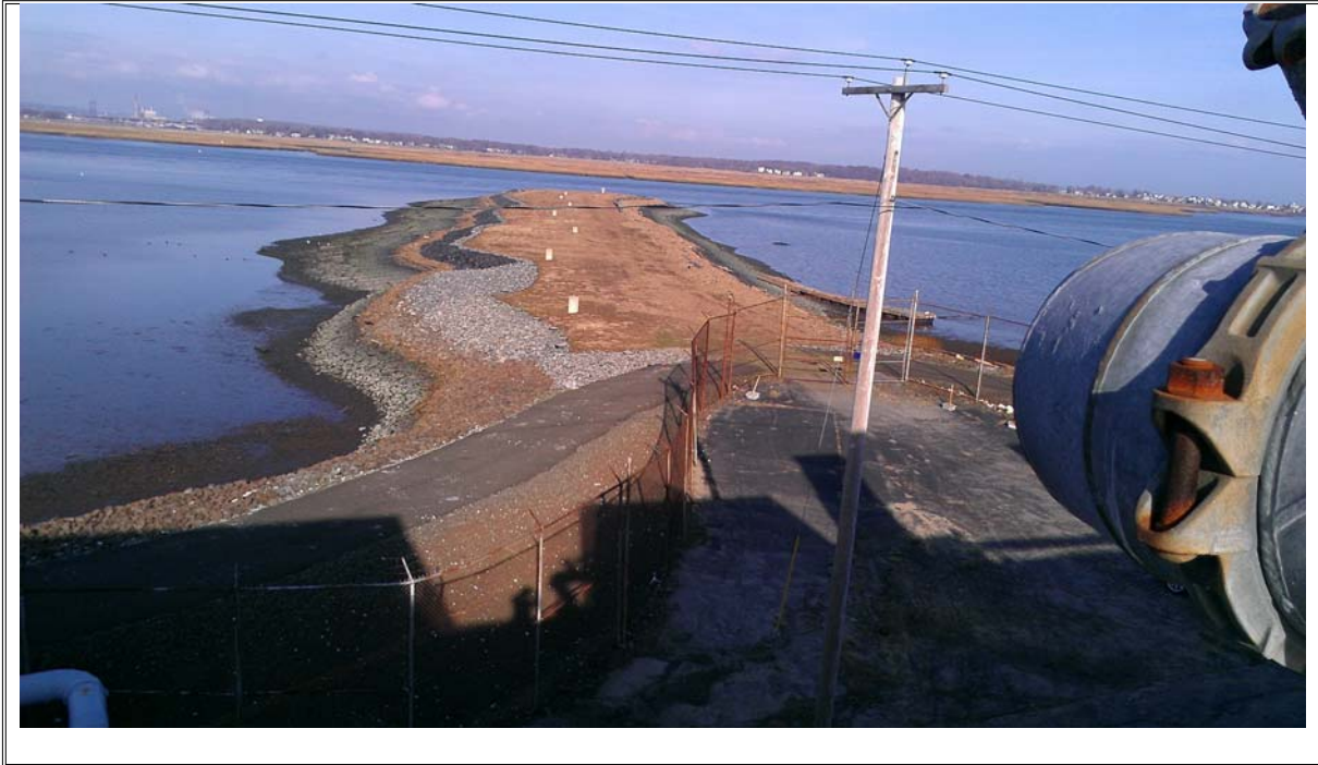
Photograph 1: Top of causeway, view to northeast
