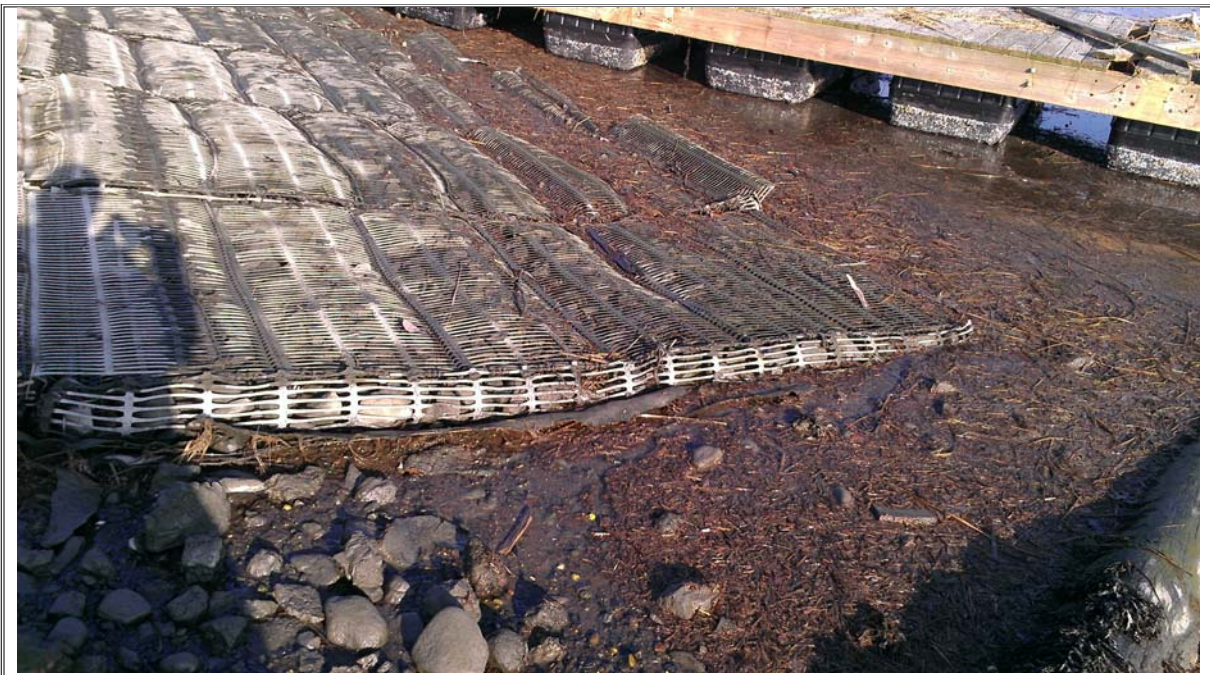
Photograph 7: Transition between upper and lower cover system, geotextile exposed adjacent to fence post base
