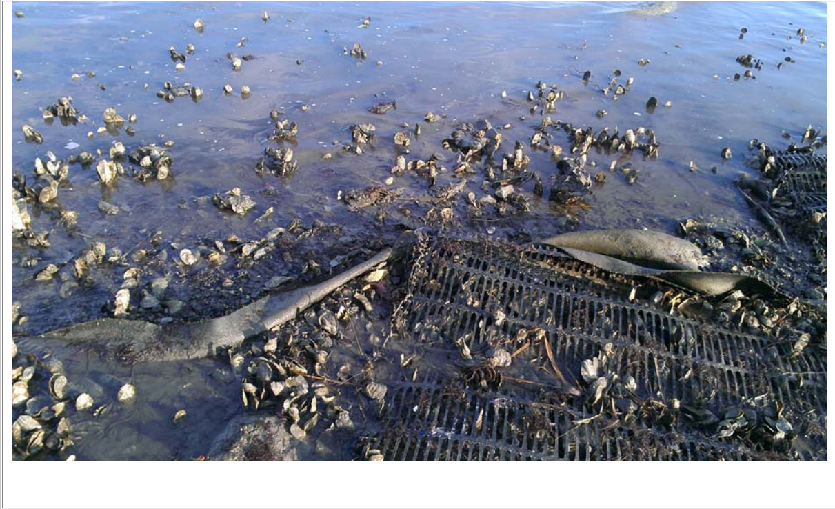
Photograph 17: Marine mat edge at northeast tip of causeway showing minor woven geotextile base exposure
