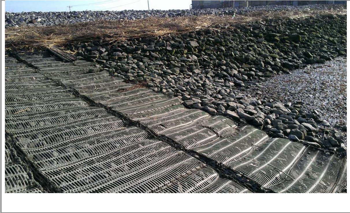
Photograph 29: Transition between marine mat and riprap slope, west face of causeway
