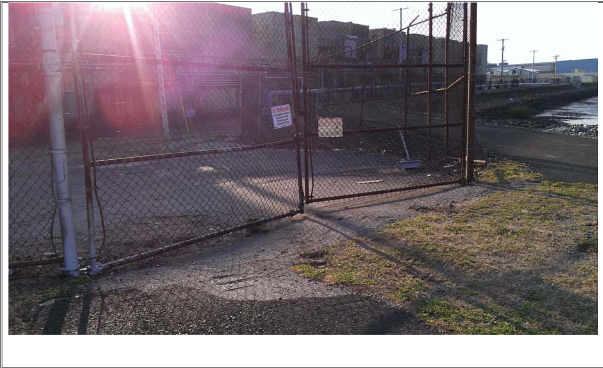
Photograph 40: View of access gate
