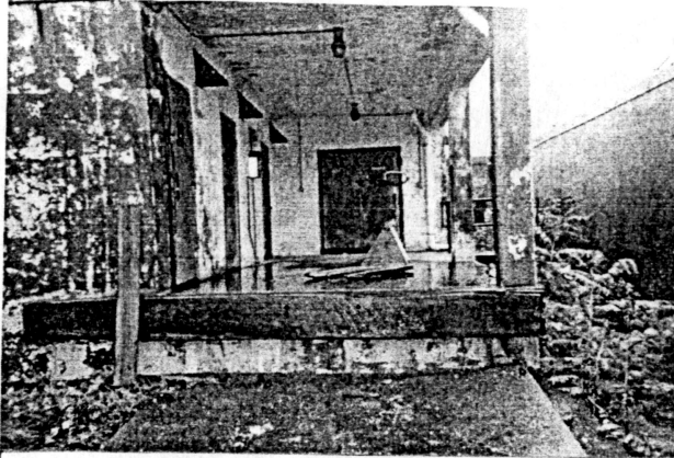
Photo 9, Emptied Loading Dock
