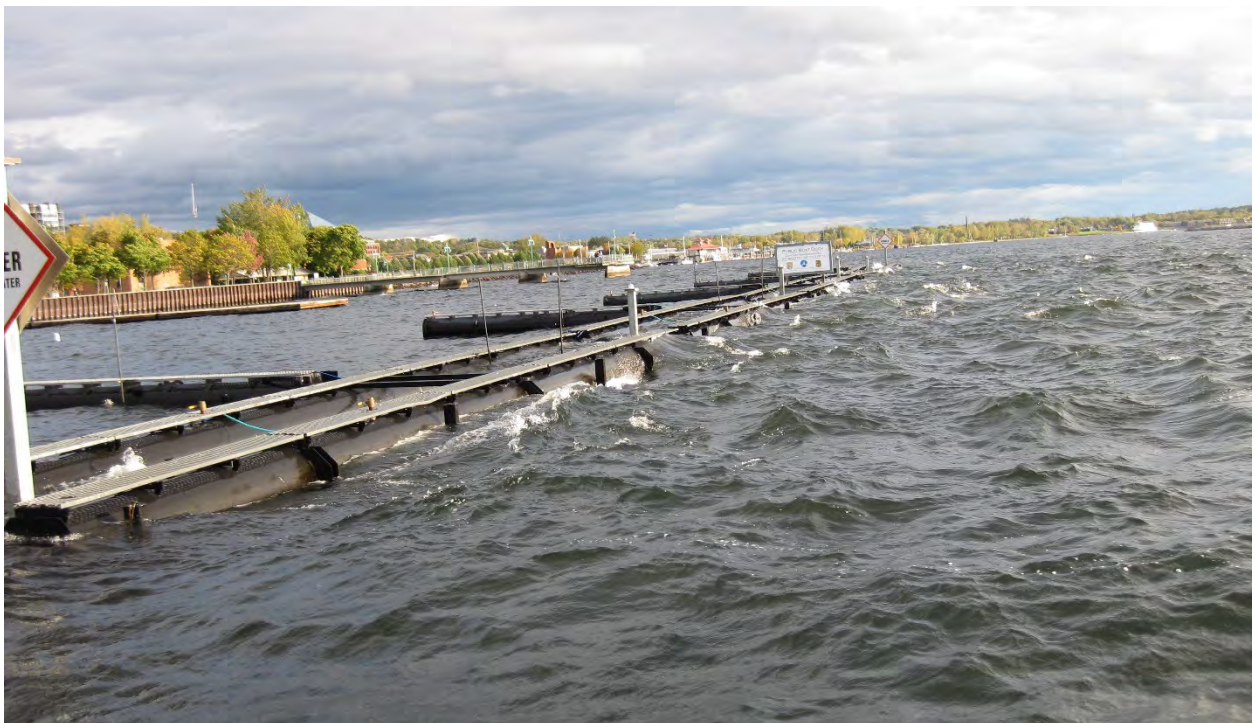
Figure 12. Engineering Control – Wave Attenuator. Source: Kropf
