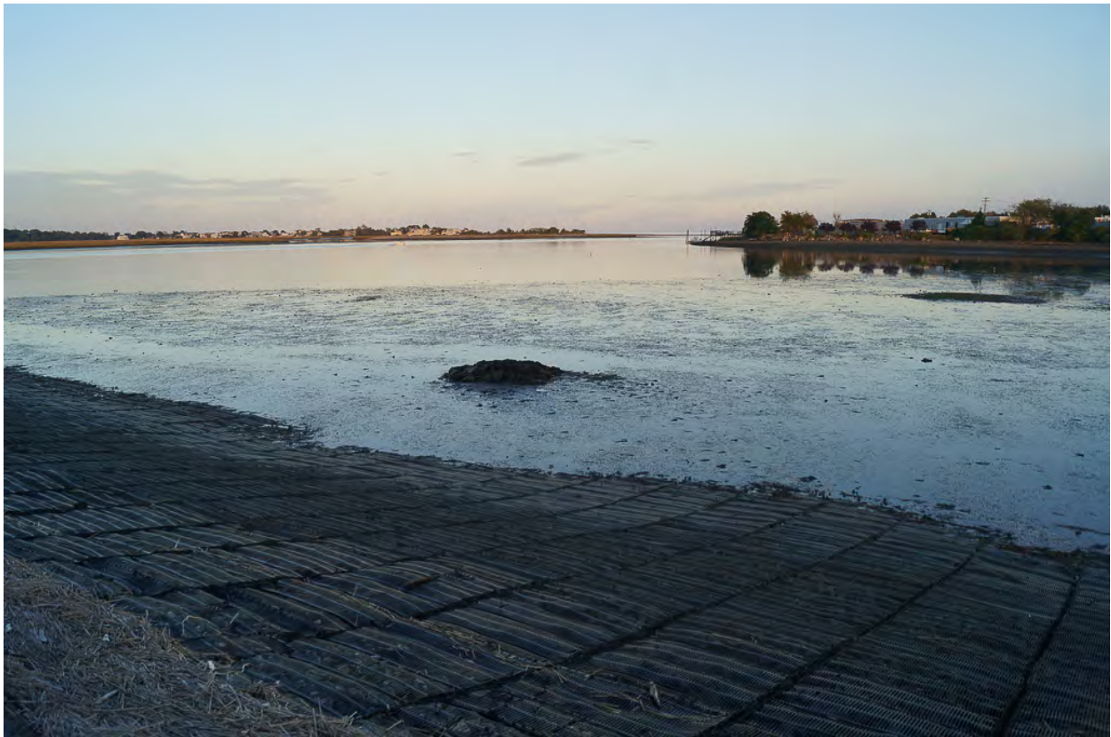
Photo 13. Mid - Causeway looking east across east tide flat, near low-tide. Note isolated debris pile (riprap). October 6, 2017.
