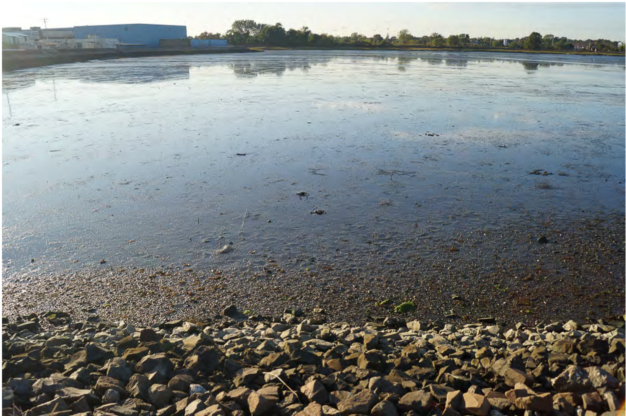
Photo 12. South Causeway on rock revetment looking west across west tide flat, near low-tide. October 6, 2017.
