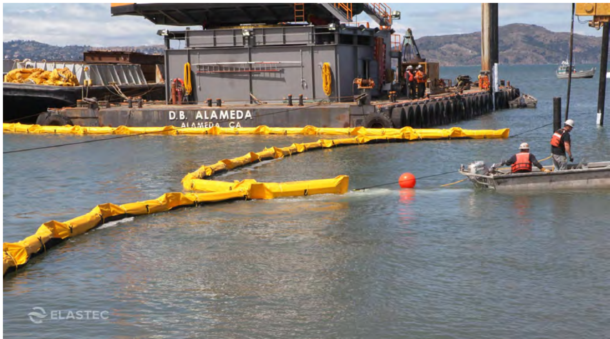
Figure 13. Engineering Control – Silt Curtain, Type III. Source: Elastec
