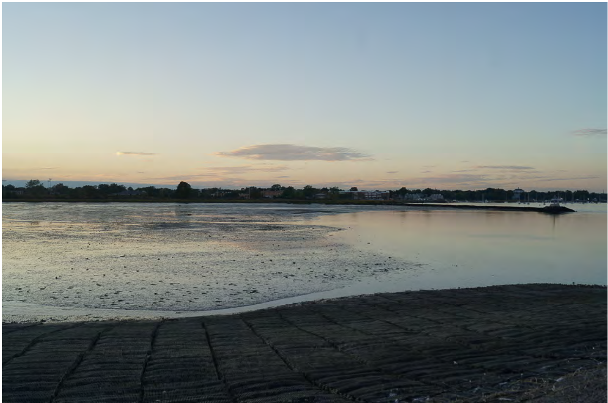
Photo 15. Mid - Causeway on marine mattress erosion control cover system looking west across west tide flat, near low-tide. Note subtidal zone. Note emergent jetty. October 6, 2017.
