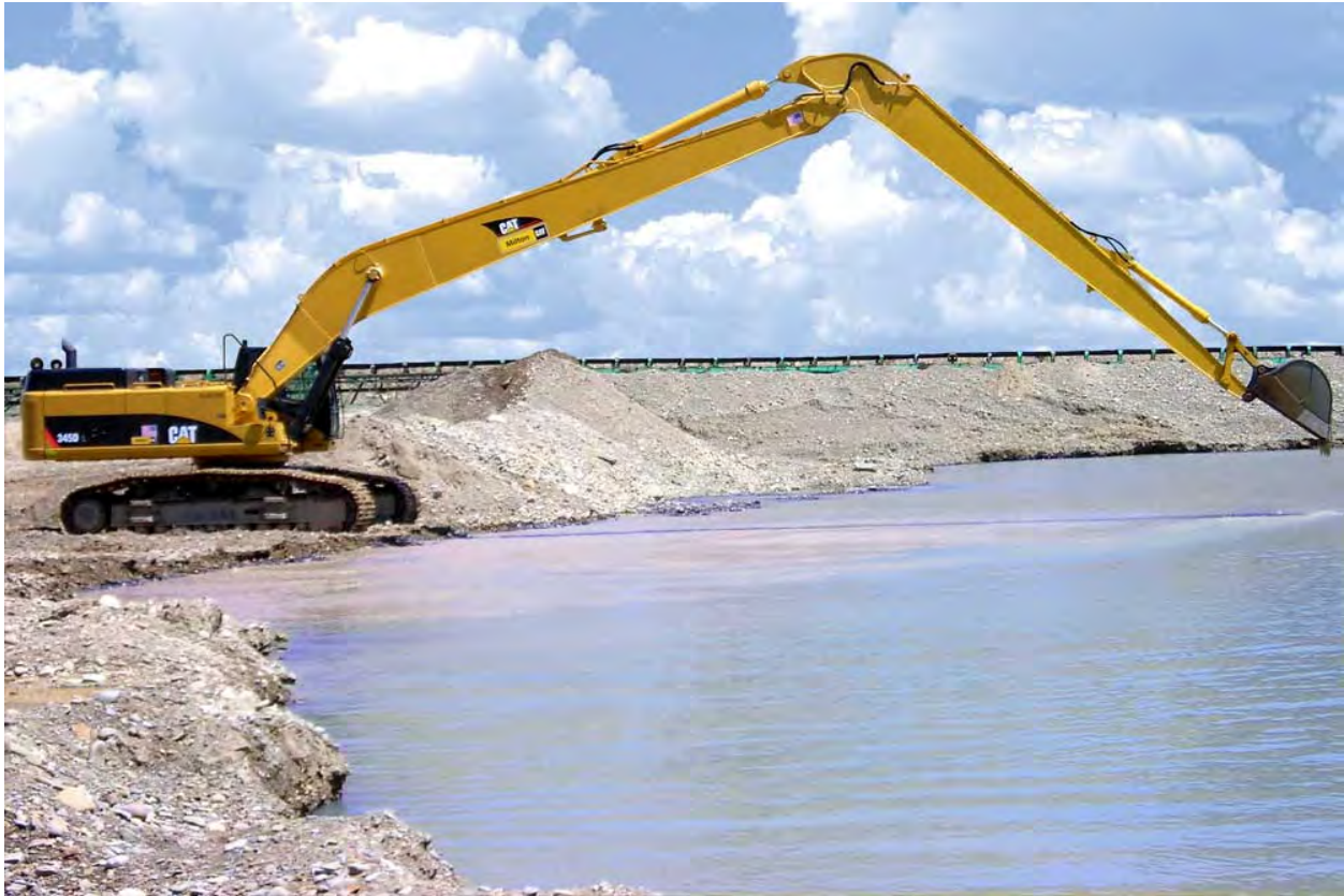
Figure 9. Alternative 5 – Long Reach Excavator. CAT 345B. Source: Pierce Pacific
