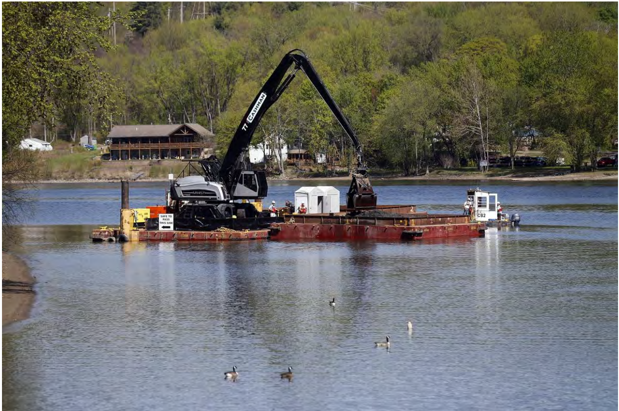
Figure 4. Alternative 2 - Precision Excavator Dredge, Shallow Draft Barge, Push Boat, Hudson River, 2013
