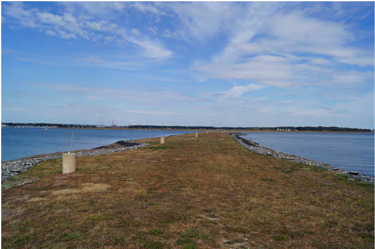
Photo 3. South Causeway, looking north, mid-tide. October 6, 2017.
