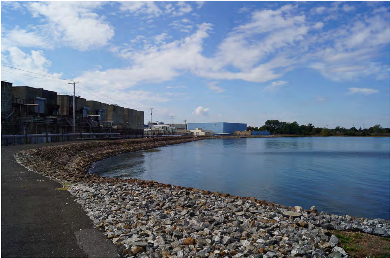
Photo 5. Head of Causeway looking west across west tide flat, dike and revetment, mid-tide. October 6, 2017.
