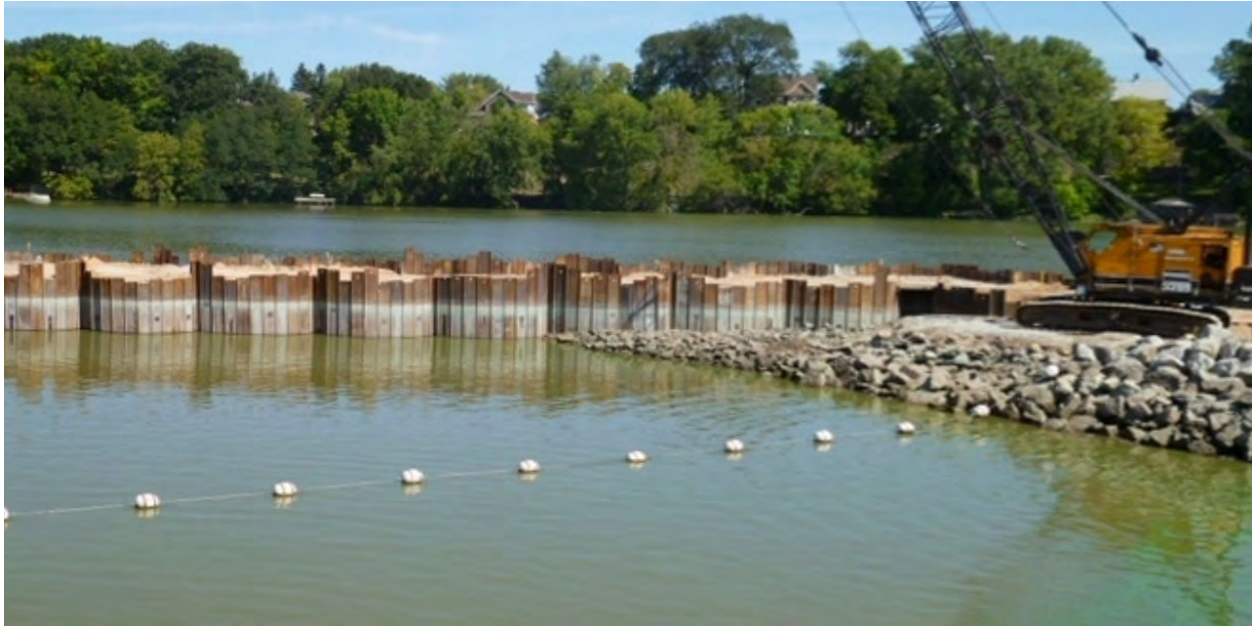
Figure 11. Engineering Control - Cofferdam. Source: Pilebuck
