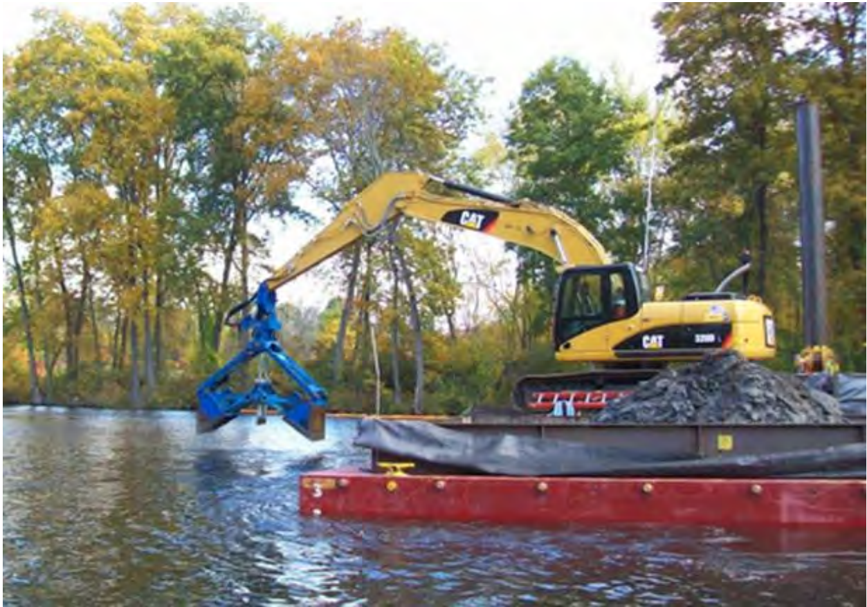
Figure 3. Alternative 2 - Precision Excavator Dredge, Shallow Draft Barge, Hudson River, NY, 2009.
