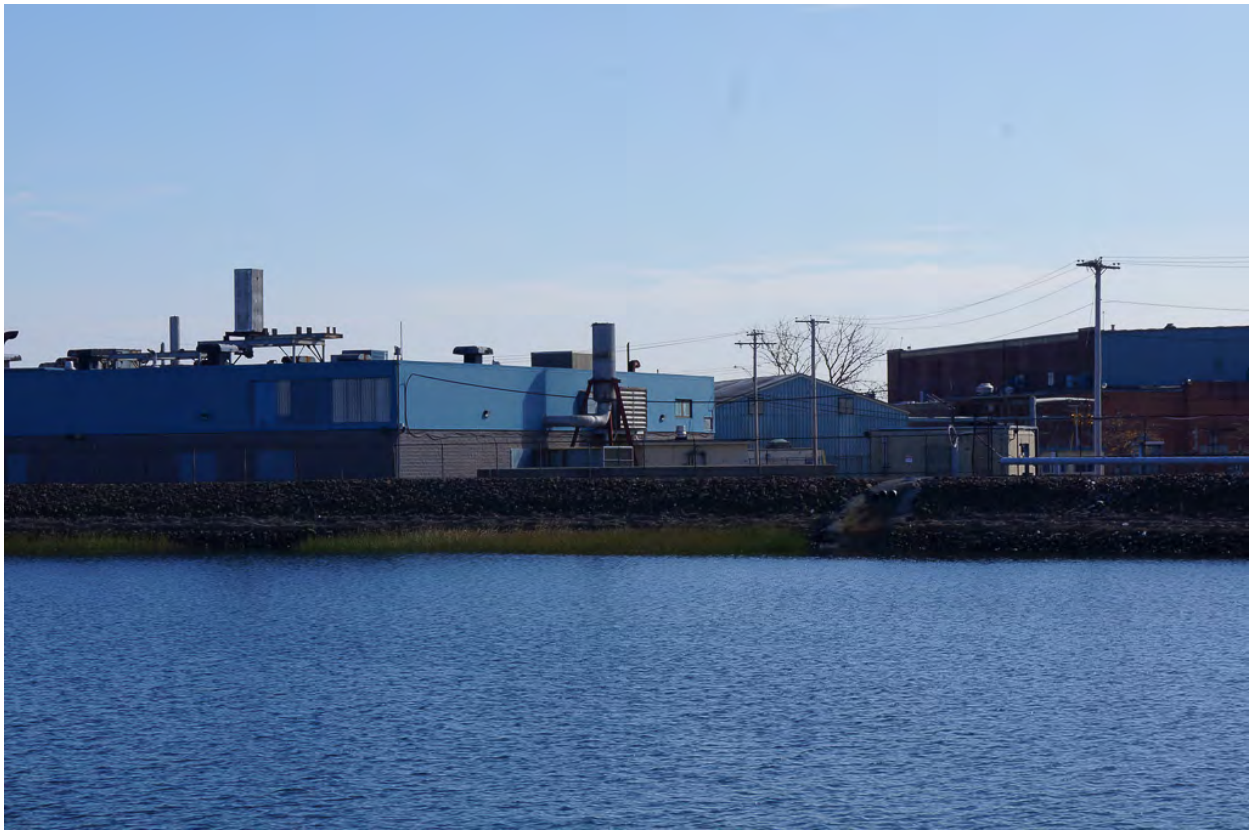
Photo 11. Mid - Causeway looking southeast across east tide flat to eastern end of dike and revetment, mid-tide. October 6, 2017.
