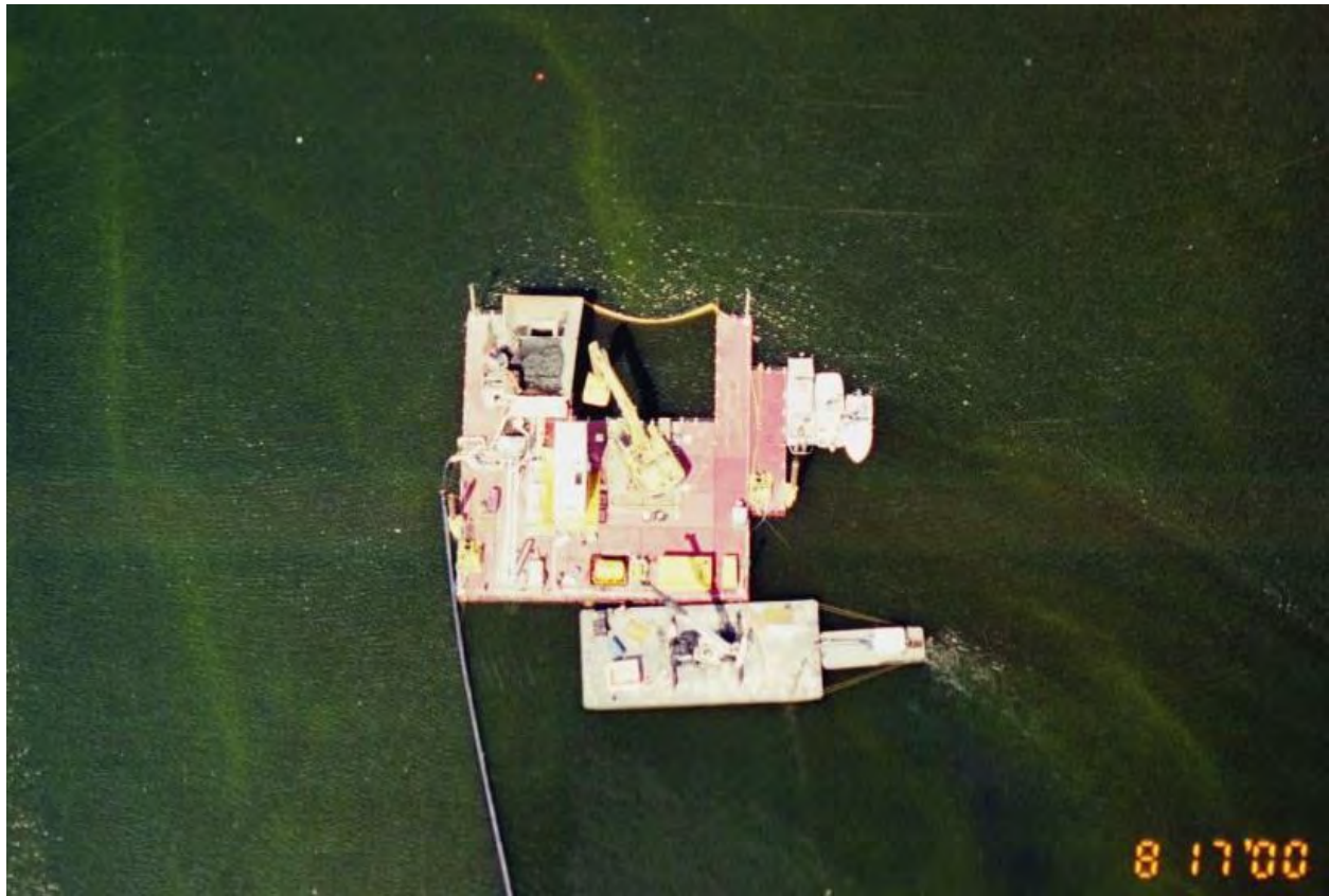
Figure 5. Alternative 3 - Hybrid Precision Excavator Hydraulic Transport Dredge, New Bedford, MA, 2000
