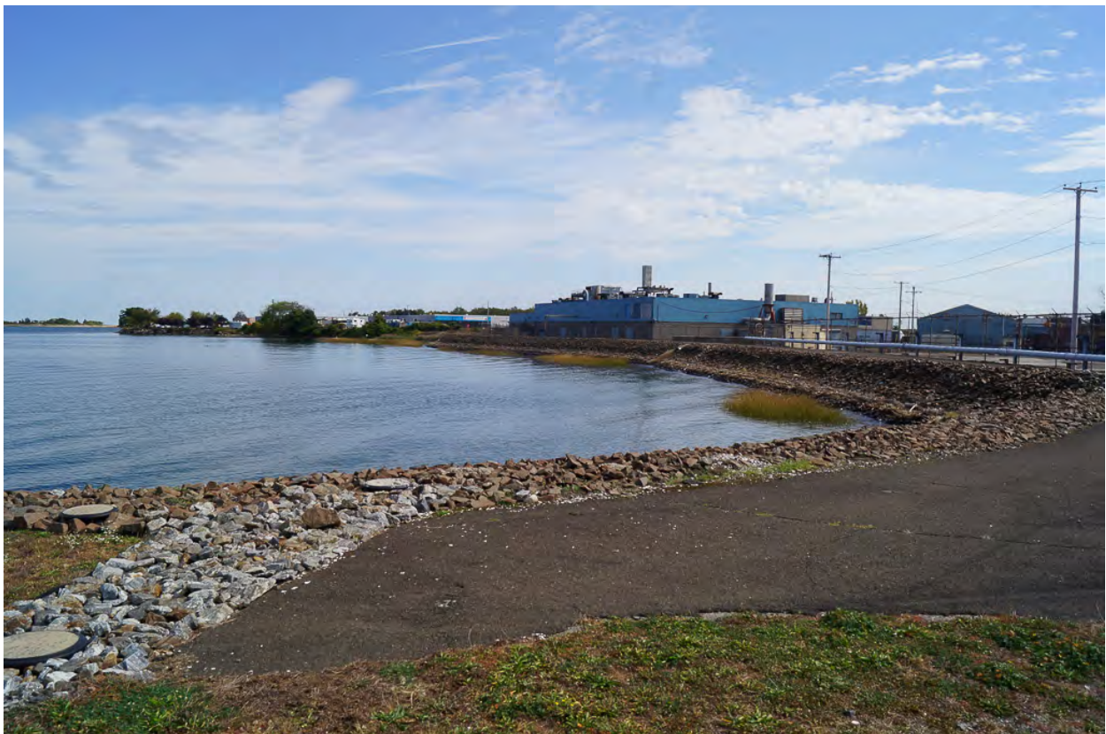
Photo 4. Head of Causeway looking east across east tide flat, dike and revetment, mid-tide. October 6, 2017.
