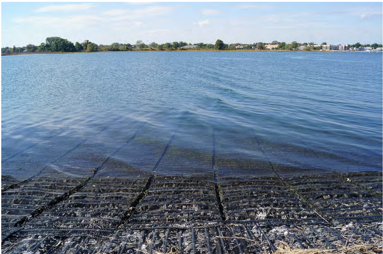
Photo 10. Mid - Causeway on marine mattress erosion control cover system looking west across west tide flat, mid-tide. Note vessel wake has approximate 6 ft. wavelength, 0.5 ft. amplitude. October 6, 2017.
